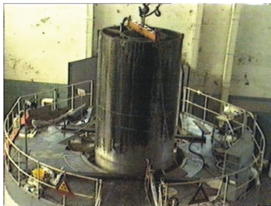
Figure 3. Lifting of the reactor vessel
