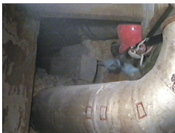
Figure 4. Dismantling of the concrete wall in the primary circuit pump house
