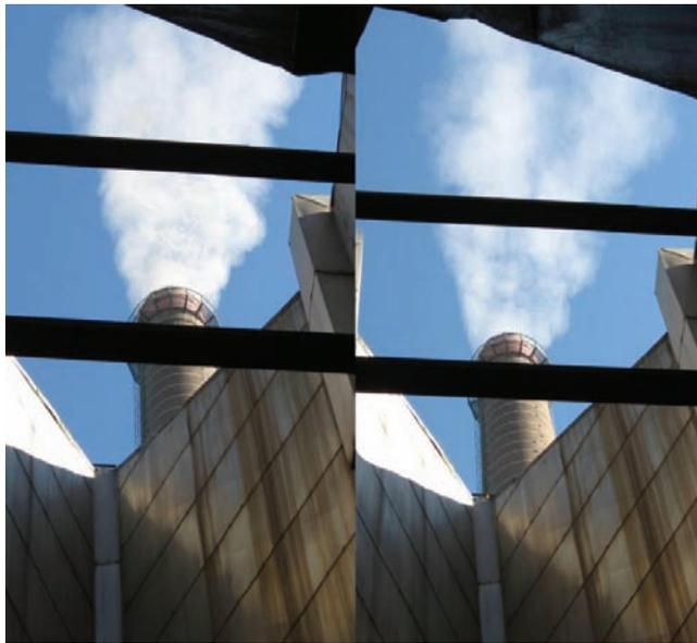
**Fig. 14** – The left part of the figure illustrates the smoke appearance in configuration of  $4 \times 50\text{Hz}$ . The right part of the figure illustrates the smoke appearance in configuration of  $2 \times 50\text{Hz} + 2 \times \text{HF}$ .
